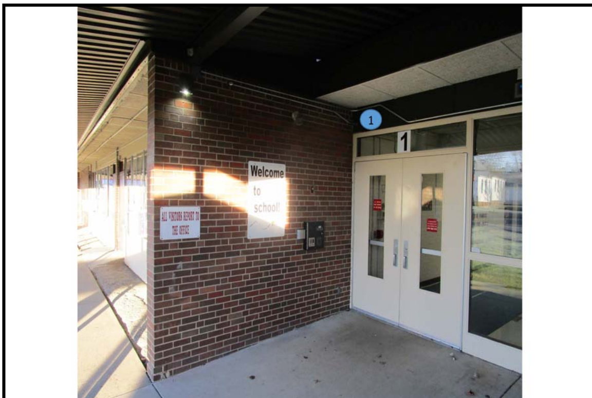
Photograph 2: Detailed view of the main entry to Andrew Heights Elementary, looking northwest.
