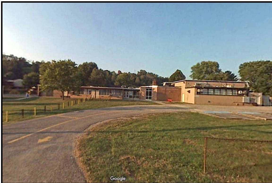
Photograph 1: View showing the south elevation of Andrew Heights Elementary, looking northeast. (Google Maps)
